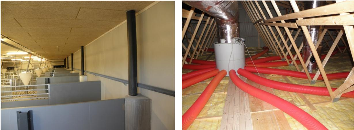
*Figure 4. Pit exhaust suction tubes between each second pen (to the left) and combining of twelve pit exhaust suction tubes to a single exhaust in the attic (to the right).*
