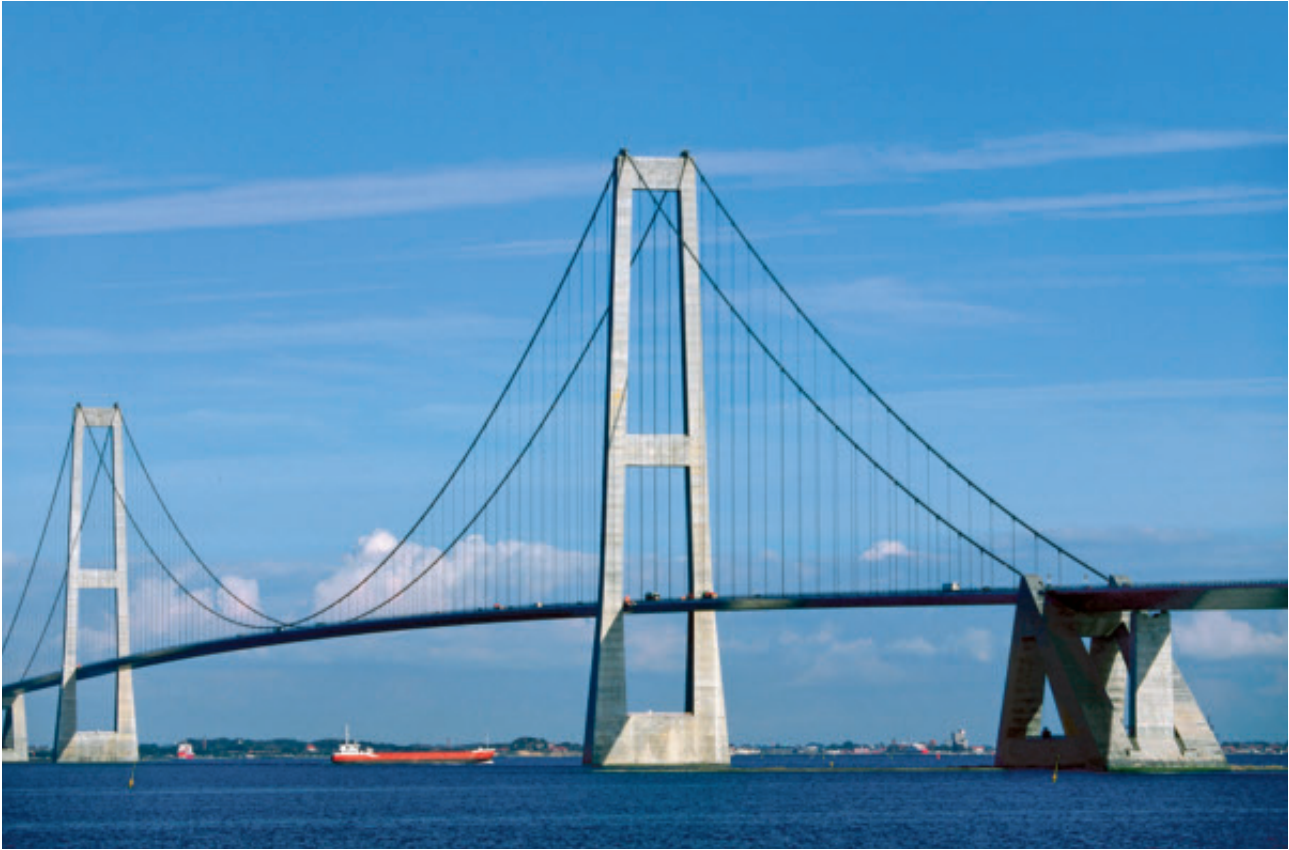
Fig. 2. The Great Belt East Bridge. (Photo: Sund & Bælt)
